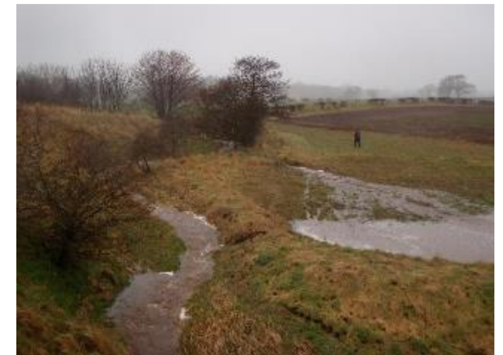
Runoff attenuation feature, Belford (source: Newcastle University)
