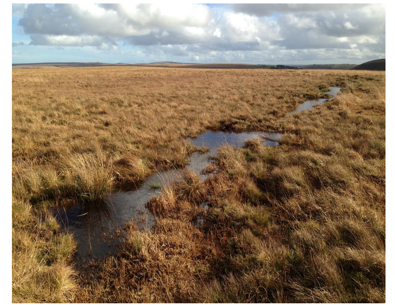
Exmoor Mire - Restored ditch showing pools formed behind peat blocks and wet areas downslope (source: Environment Agency)
