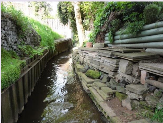
Looking for hazards along the Wesley Brook (Photo: Colin Dalziel, SFPG)
