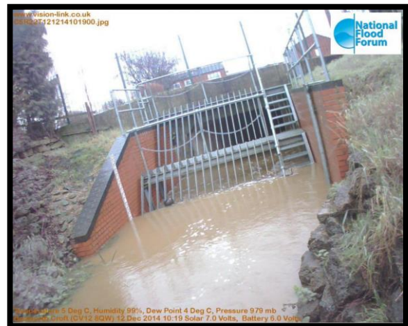
An image of the CCTV footage that the Bedworth group are using to monitor blockages at the trash screen.
