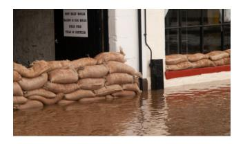
Sandbag walls have been traditionally employed as demountable flood walls but they have a detrimental effect on the environment with the need for transporting and dredging sand and associated carbon dioxide emissions. They require sig-
