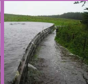
Permeable timber barriers (below and below left).
